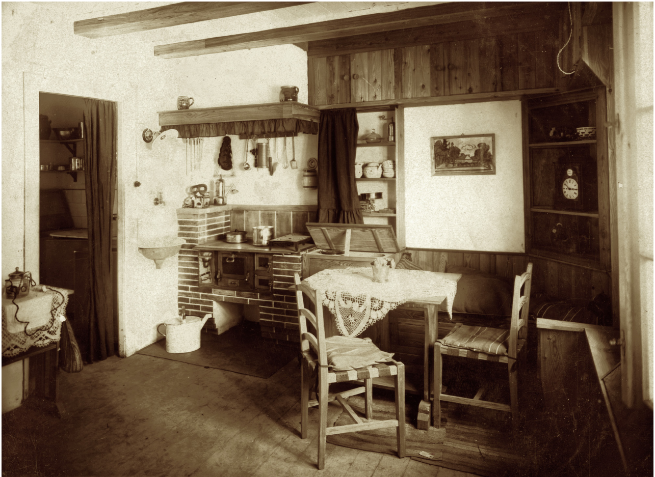
Figure 5: Live-In Kitchen, First Stage of Construction, Core-House Type 7, Shown at 'Small Garden, Settlement and Housing Exposition,' Vienna, 1923. Photographer: Joseph Perscheid, Vienna. Source: Schütte-Lihotzky Inheritance, University of Applied Arts Vienna, Collection and Archive, PRNR 34/19/FW.
