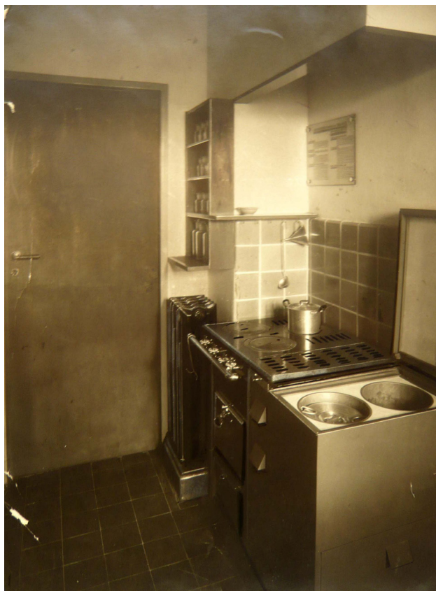
Figure 8: Frankfurt Kitchen, Stove Complex with Hay Box (On the Far Right), Frankfurt, 1927. Photographer: H. Collischonn, Frankfurt. Source: Schütte-Lihotzky Inheritance, University of Applied Arts Vienna, Collection and Archive, PRNR 50/15/FW.
